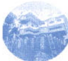
Loans for House Repairing
